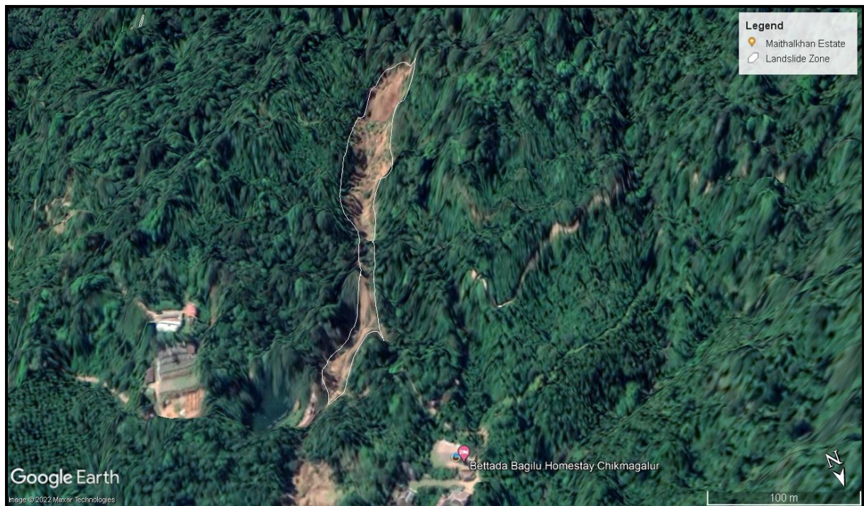
Figure 43: Major Hulikatte landslide from Google image
