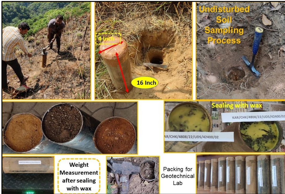
Photo 3: Field photograph showing sample collection, packing, weighing, and sealing of cylinder sample tubes.
